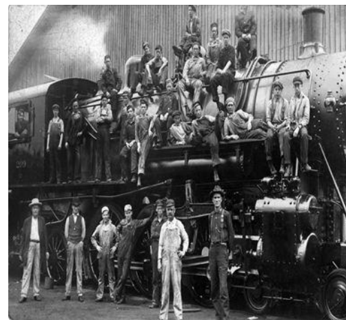
Decatur Railroad Shop
