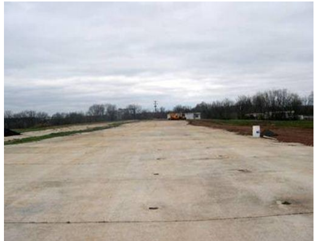
Highway 20 DMAC Field
