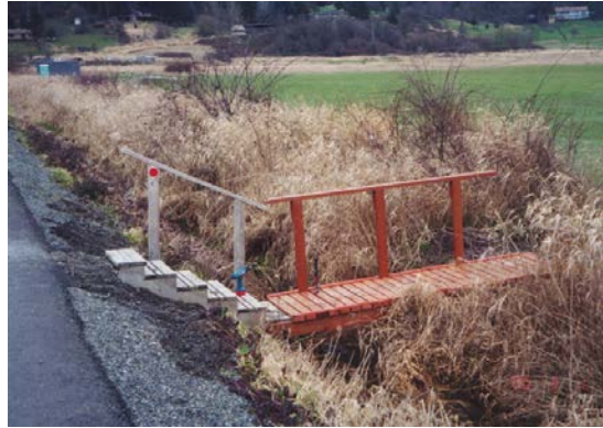
Bridge over drainage ditch, built by Hinze for his club. It was used for crossing 116 th street from the soccer fields to “60 Acres South” field in the winter.
