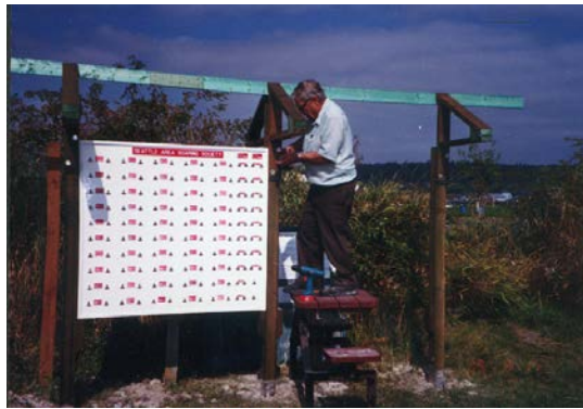
1999: Assembling the North frequency board
