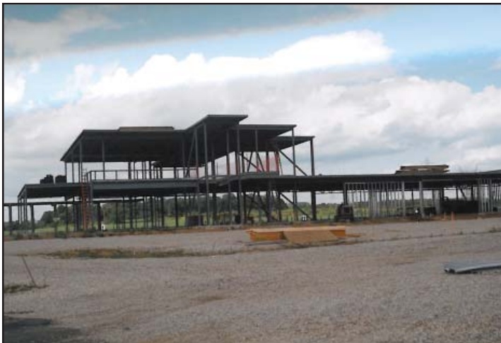
The early stages of construction. National Model Aviation Museum photo.
